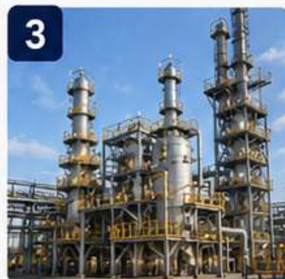
3 SULPHUR RECOVERY UNIT (CLAUS PROCESS)
